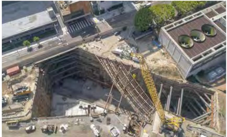
control vertical movement of the system. Prior to the installation of the unpinning, liquid levels, crack gauges, and monitoring points were affixed to the basement structure. However, no measurable movement or cracking of the basement structure has been observed. Figure 12 includes a photograph of the completed underpinning system a sketch of the final underpinning design.
